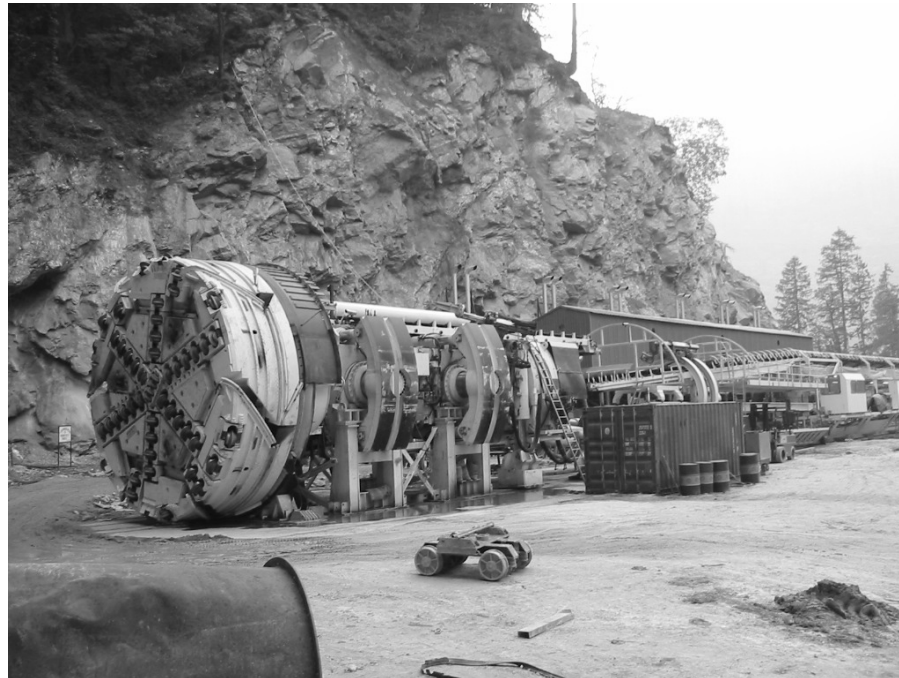
Photograph 1 Open mode TBM assembled outside Adit-II
