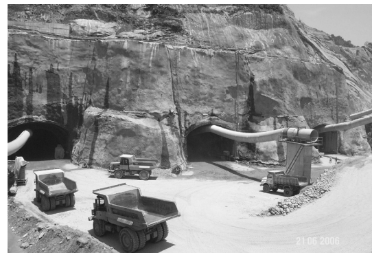
Photograph 4 Outlet portals of Diversion tunnel
